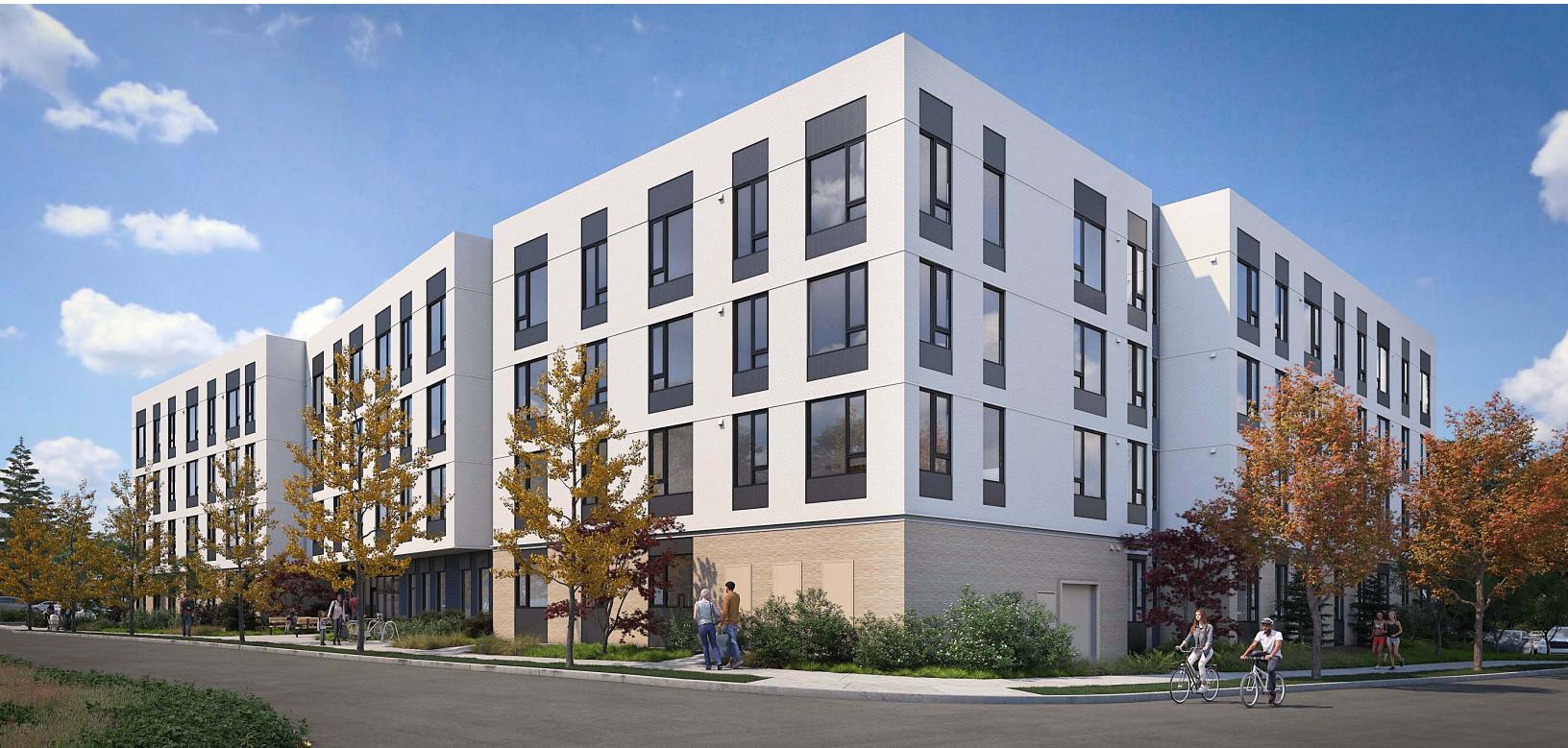
Located in the Aloha community in Washington County, Oregon, Cedar Rising provides 82 permanent affordable apartments for families.
