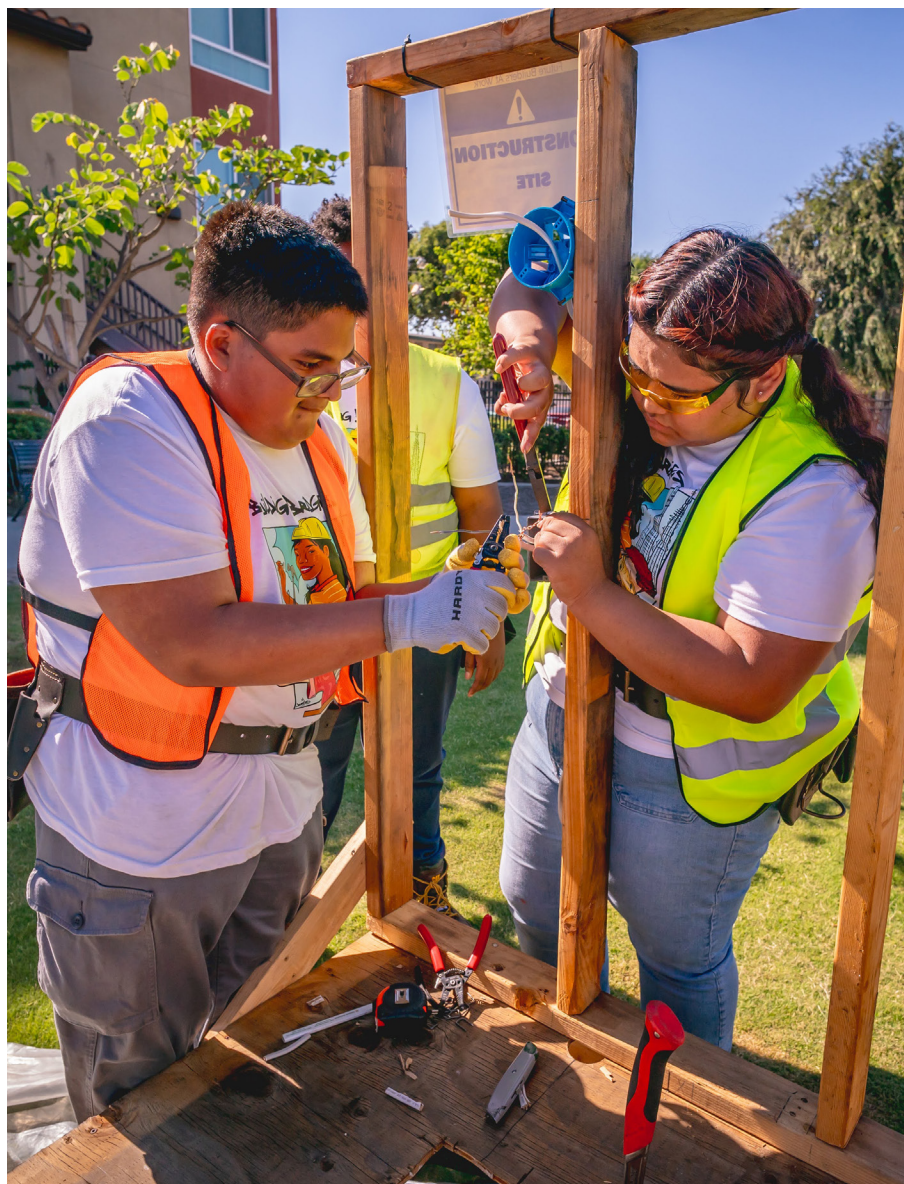
Young Jordan Downs residents learn skilled trades through the two-week Building Bridges Program, a partnership with Harbor Freight Tools for Schools
