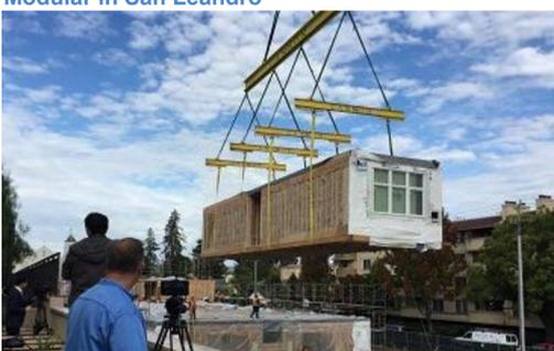
Construction of San Leandro Senior is progressing quickly, as Cannon Constructors North is working with Guerdon Modular Buildings to crane 109 factory-built modules into place on the concrete podium. BRIDGE estimates that the modular process will trim a projected 22 weeks off the construction schedule. The 85 new apartments for low-income seniors are expected to be complete in mid-2018. [Read more.](#)
